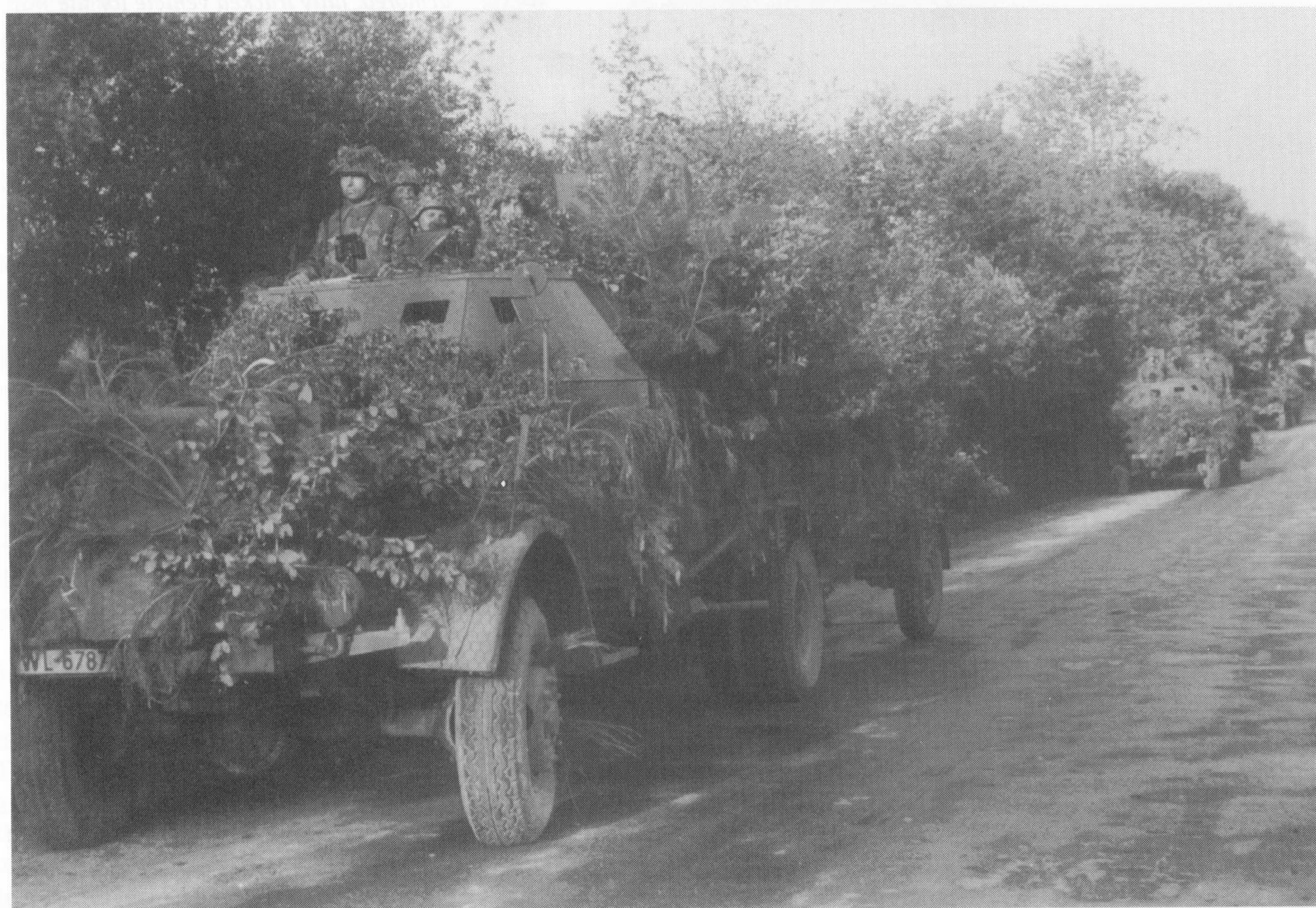
A battery of 20mm Quadruple Flak on the march. The guns are mounted on lightly-armored, camouflaged 4.5-ton trucks. Sonderanhänger 36 trailers contained the crew's equipment as well as ammunition for the guns.
