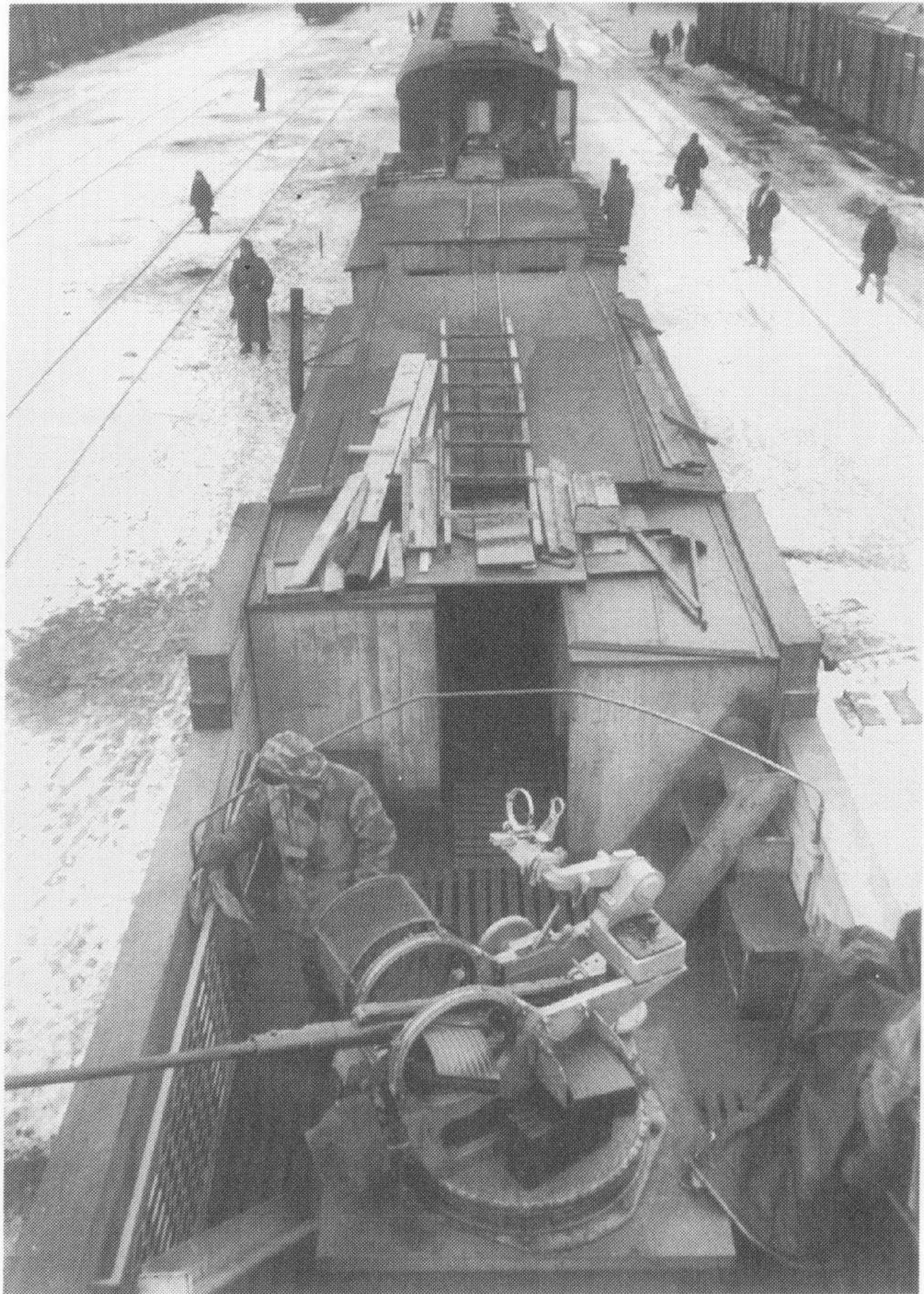
Above: A view of Light Flak Gun Car I (E), armed with a 20mm Flak 38. The gun mount was bolted to the wooden platform of the gun car. Clearly visible is the barrel deflector frame, which prevented the gun from hitting the cars in front with its fire. To the right and left of the entrance to the crew living quarters are shelves for storing accessories and a quantity of ammunition. The double-walled sides protected the crew from fragments. The space between the walls was filled with iron-reinforced concrete. The ladder lying on the roof of the living quarters was leaned against the side of the car for the crew to climb down. It was planned to install wooden steps inside the car for this purpose.
